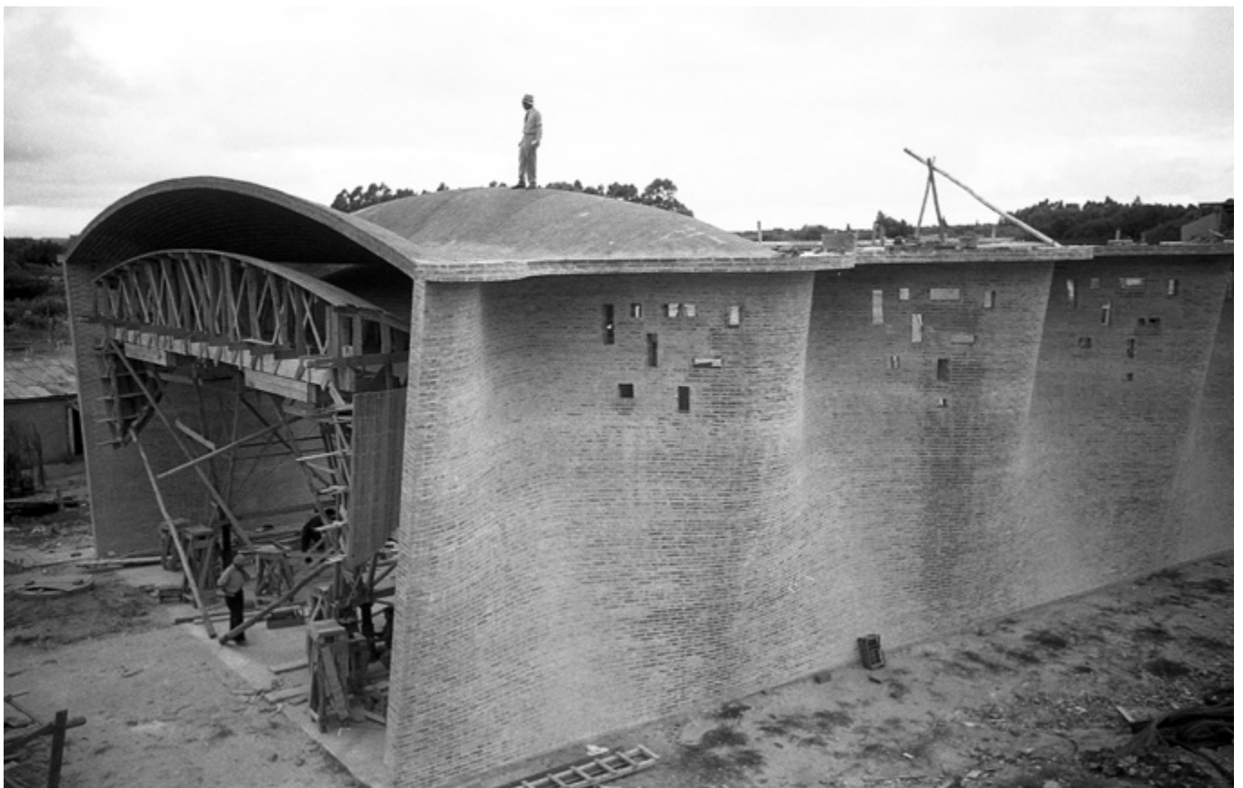
Fig. 2. Church of Christ the Worker, Atlántida, Uruguay, 1958. Eladio Dieste on the roof, watching the dismantling of the scaffolding of the first section of the vault. Dieste & Montañez S.A. Photographic Archive, Dieste Foundation.
