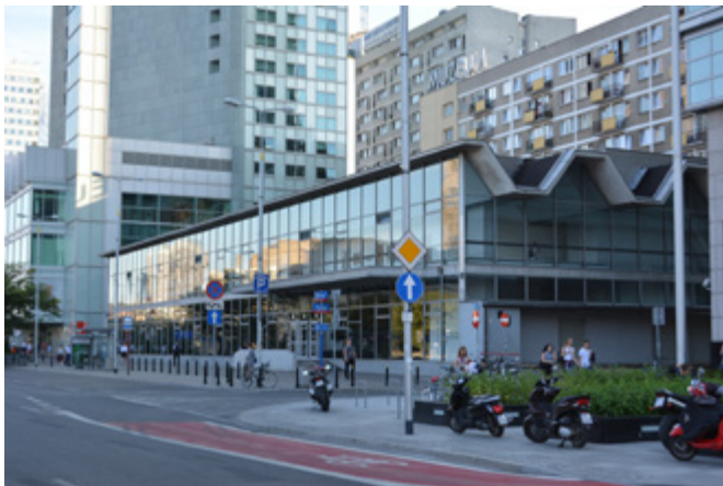
Fig. 3. “Emilia” pavilion, where the Museum of Modern Art in Warsaw was operating in 2012-2016 (afterwards it was dismantled). It is surrounded by socialist residential blocks and modern office buildings. Opposite, across the street, is the Palace of Culture and Science. (Figs. 3-6 © Author).
