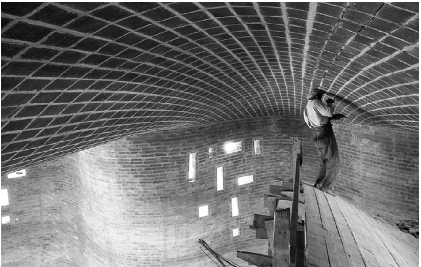
Fig. 3. Church of Christ the Worker, Atlántida, Uruguay, 1958. Mason filling brick joints of the vault. Dieste & Montañez S.A. Photographic Archive, Dieste Foundation.
